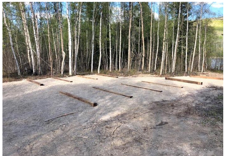
6x6 foundation layout for Sea can Storage units. Lumber foundation built on gravel pad. Gravel pad constructed by W6 Contracting. Gravel pad promotes drainage, prevents vegetation growth and provides clean work area. May 2020
