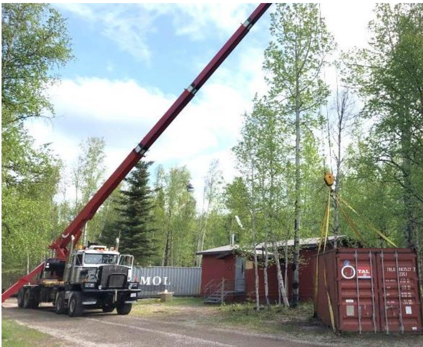
Crane moving existing 20' Sea can to new foundation. Grey 40' Sea can shown behind crane. May 30, 2020
