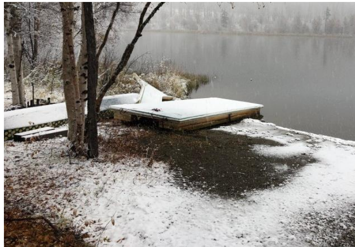
Moved dock out of water for winter to prevent damage from ice. Installed anchor floats and stored chains. October 2020
