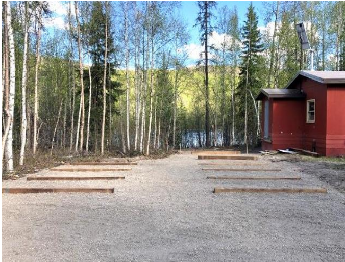
Constructed foundation for Sea can Storage units with 6x6 treated lumber. Foundation was built so each unit is square and level with one another. This will allow for easy construction of roof structure at some point in future. May 2020
