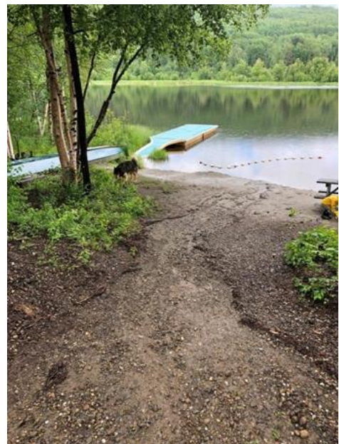
Installed Dock for summer. Maintenance of drainage swale to prevent erosion of beach area. Drainage was full of leaves and gravel. Repaired eroded area and raked beach area. May 2020
